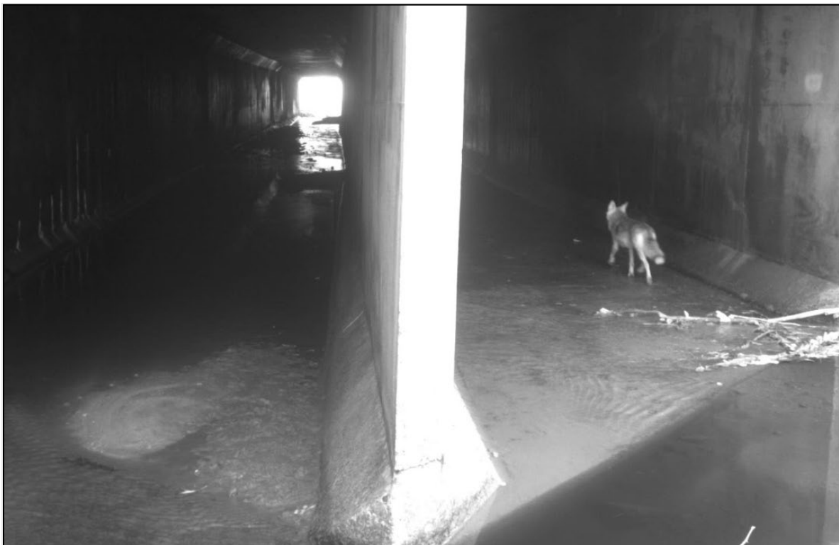
Cove Creek double box culvert, coyote. (Albemarle County)
